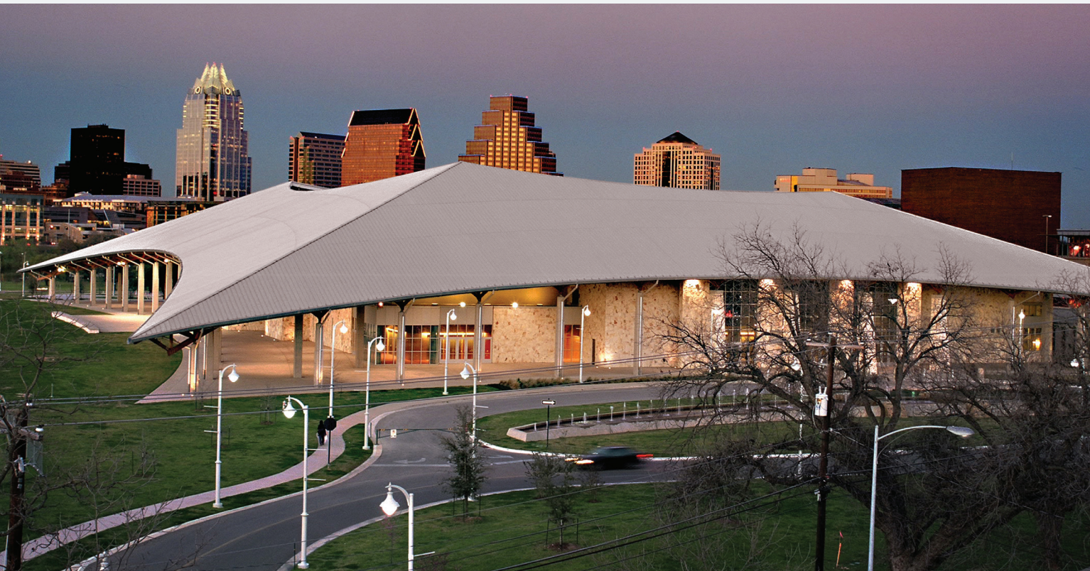
PROJECT: Lester E. Palmer Events Center LOCATION: Austin, TX PANEL PROFILE: SuperLok™ COLOR: Galvalume Plus®
